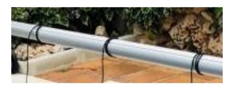
Fix the cover to the reel using 3 straps in addition to the ones used to fix the cover to the ground. VERY IMPORTANT: adjust exactly the same measure in all three, to obtain a parallel movement. If the reel goes across, adjust the measurements of the belts.
